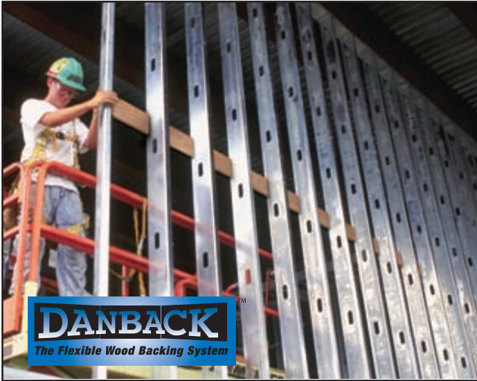
SNAP the Starter Edge into the open side of the flange
