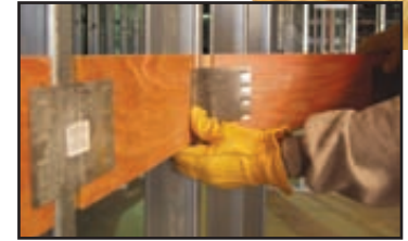
FLEX around stud flange using the flexible connector plate
