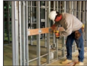
SCREW each plate to the stud flange using two small pan or wafer head screws
